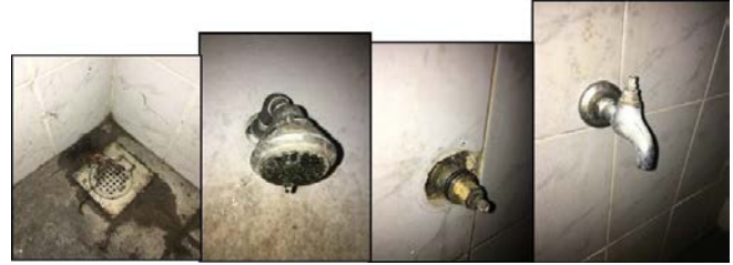
Fig. 1. Blockages, Leakages and Damages
