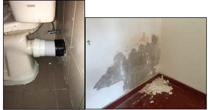
Fig. 2. Leakages
